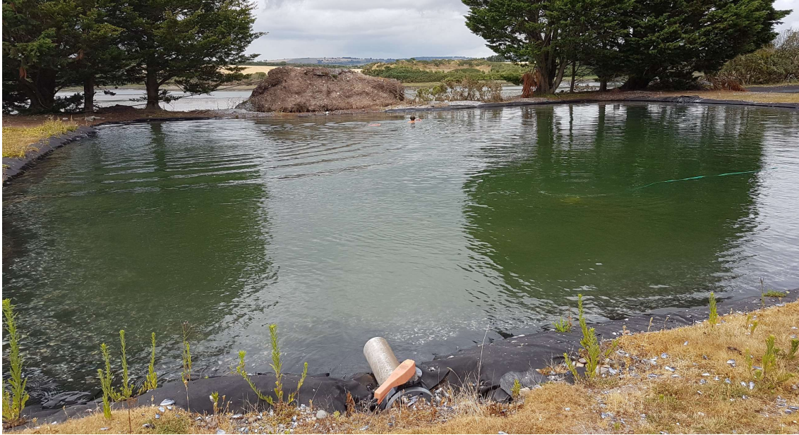
Figure 1. Oyster spatting pond in Rossmore, Ireland. The pond is located close to the sea, lined with butyl rubber and has an inlet for water. Picture Åsa Strand
